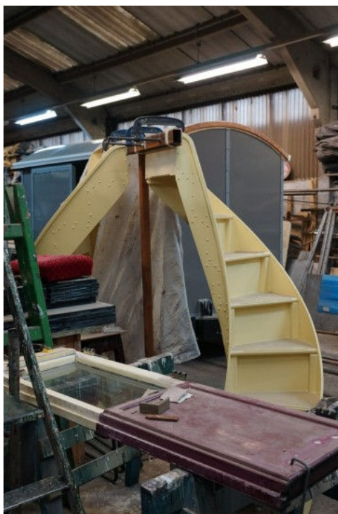
One of the staircases under attention. (All Photos: David Mee)
